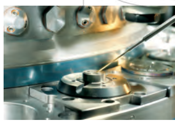
Inclined deep-hole drilling from above
